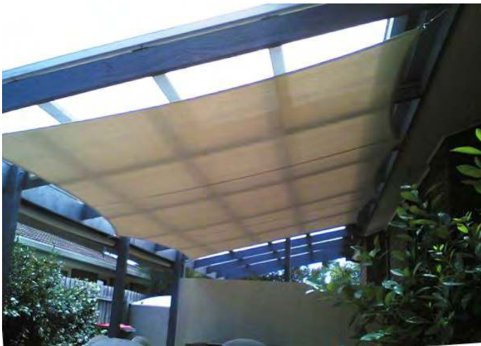
Shade sail under glass roofed pergola
